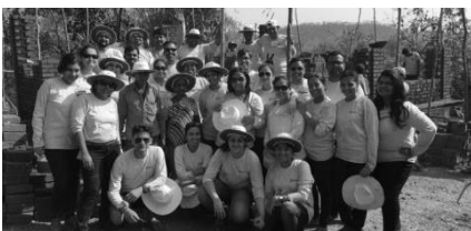
Employees volunteer in Habitat for Humanity's Build programme in a village near Karjat
